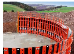
circular wall formworks
