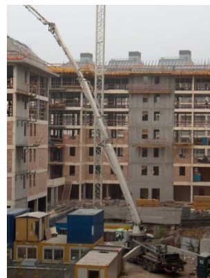
with concreting pump
