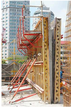
girder wall formwork system
